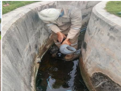
Dokumentasi Outlet IPAL PLTP (Black Water)
