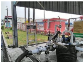
Pemasangan TSI (Tank Slide Indicator) di Shelter FAME FT Cikampek
