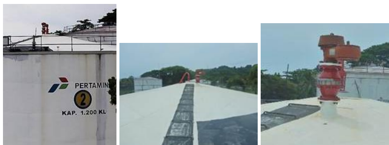
Gambar 18 VAPGUARD: Vapor Guarding System through Pressure Vacuum Valve Implementation
