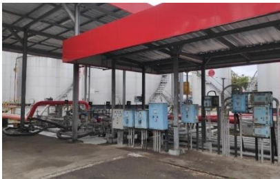
Jaringan Per-Pipa Base Oil dan Unloading Additives
