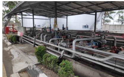
Jaringan Per-Pipa Base Oil dan Unloading Additives
