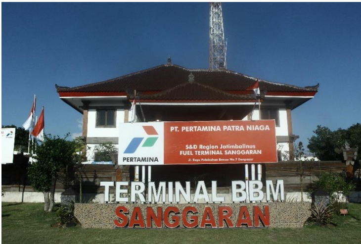
Gambar 13. Fuel Terminal Sanggaran
