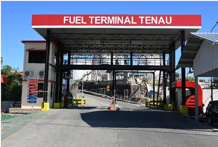
Gambar 7. Fuel Terminal Tenau
