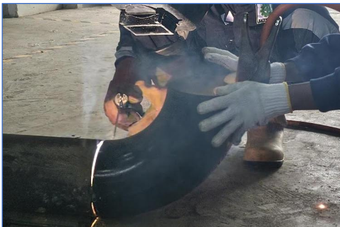
Gambar 1. 6 Proses welding pipa 6 inchi + elbow di workshop internal PGE Karaha
