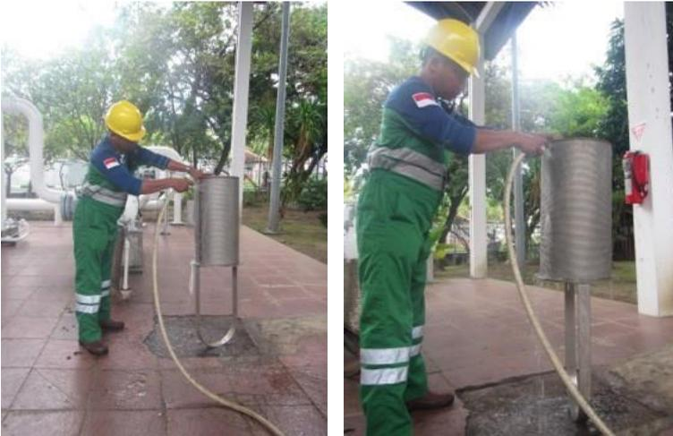
**Gambar.** Pencucian Bucket Strainer secara Manual
