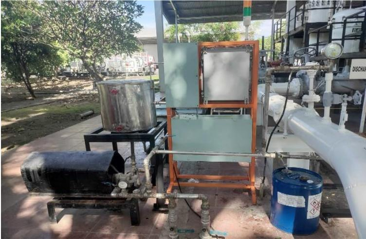
**Gambar.** Static Disipator Injector
