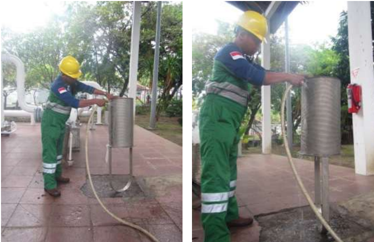
Gambar. Pencucian Bucket Strainer secara Manual
