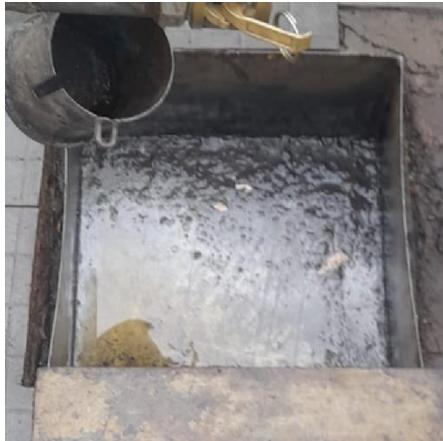
**Gambar 4.8 Bak Penampung (*Secondary Containment*)**
