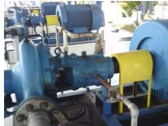
**Gambar 1.1 Pompa Booster (TOP)**
