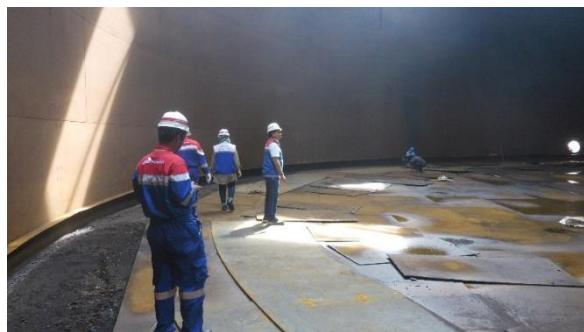
**Gambar 6.1 Korosi Dinding Dalam Tangki Timbun**
