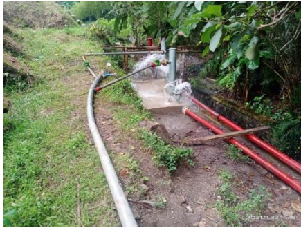
Gambar 1.1 Tampak Samping Pompa Hidram “ Green Hydrant Pump ”
